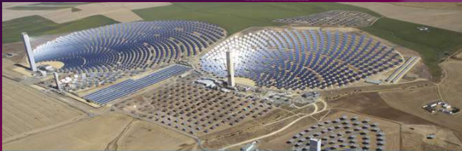
10MW + 20MW solar tower receivers, Spain
