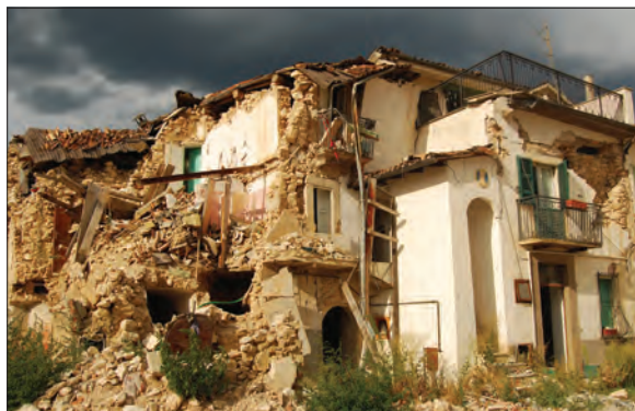
Big impact Building damage in the village of Onna, near L'Aquila in Italy, caused by the April 2009 earthquake.
