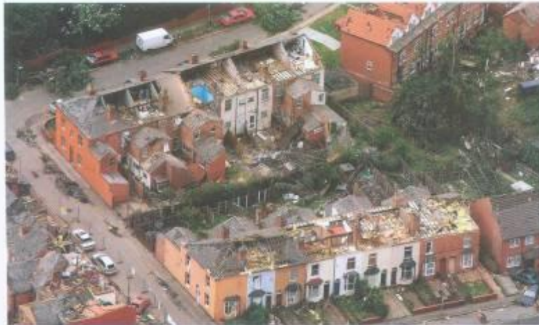
Figure 2.2 Photograph showing considerable damage to houses caused by a tornado in an area of the UK's second largest city, Birmingham, in July 2005.
