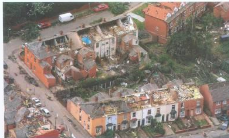
Figure 2.2 Photograph showing considerable damage to houses caused by a tornado in an area of the UK's second largest city, Birmingham, in July 2005.
