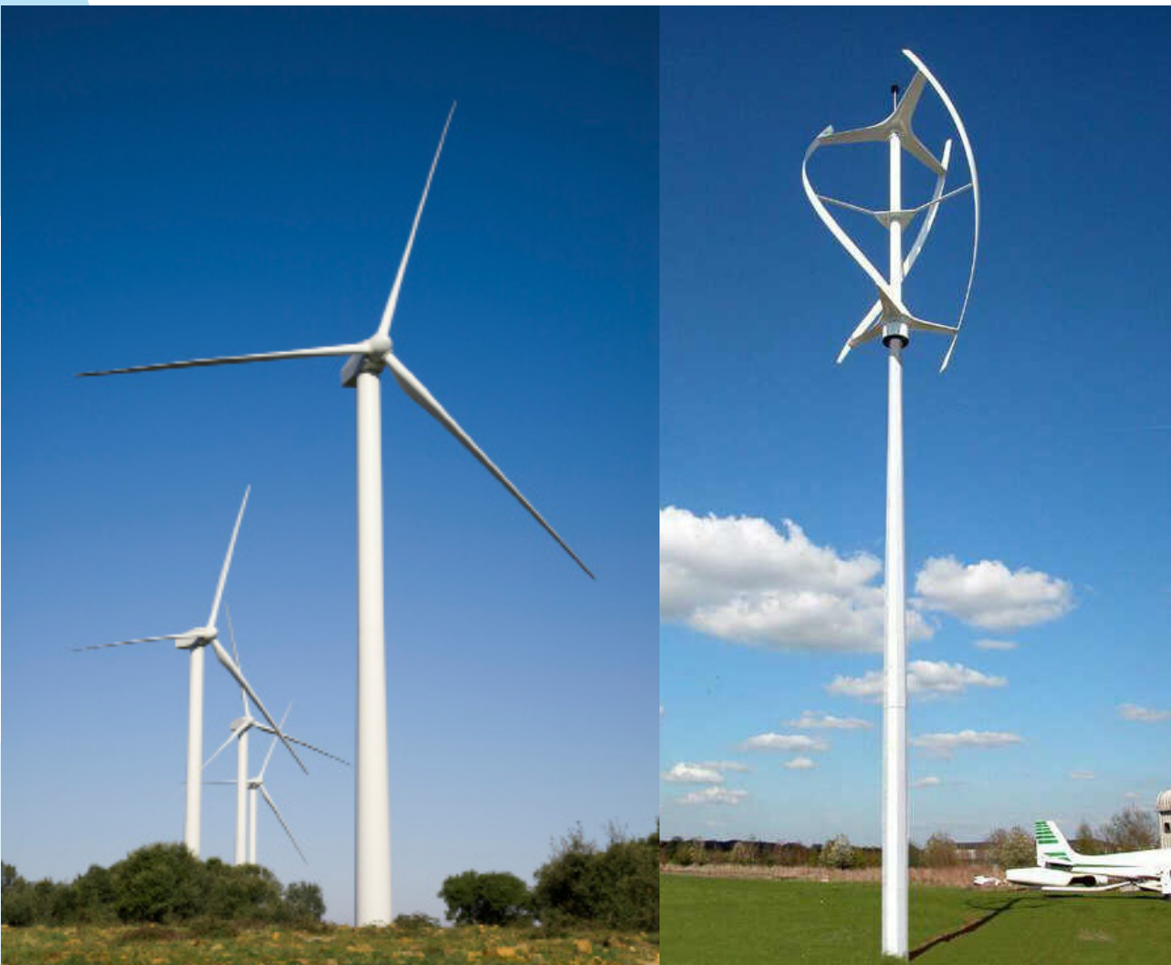
Figure 3-8. Horizontal and Vertical Wind Turbine Configurations
