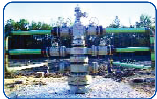
Figure 6-5. Wellhead above hydrogen cavern and integrated cavern support equipment
