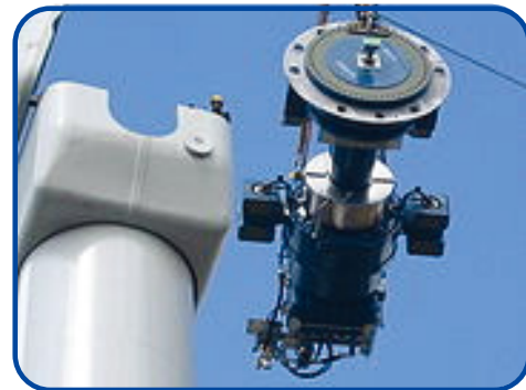
Figure 3-11. Typical components of a wind turbine (gearbox, rotor shaft and brake assembly).
