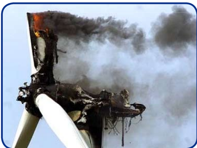
Figure 2 – Wind Turbine on Fire
