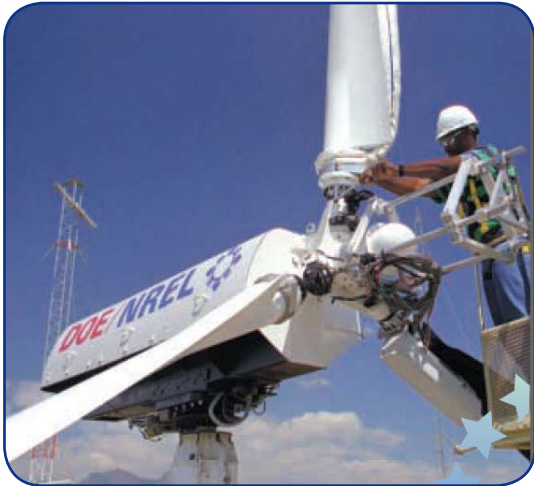
Figure 2 – Checking Turbine Blades for Stress
